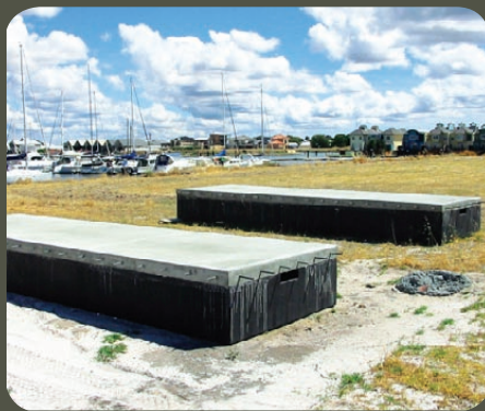
Walkway pontoons ready for timber whalers
