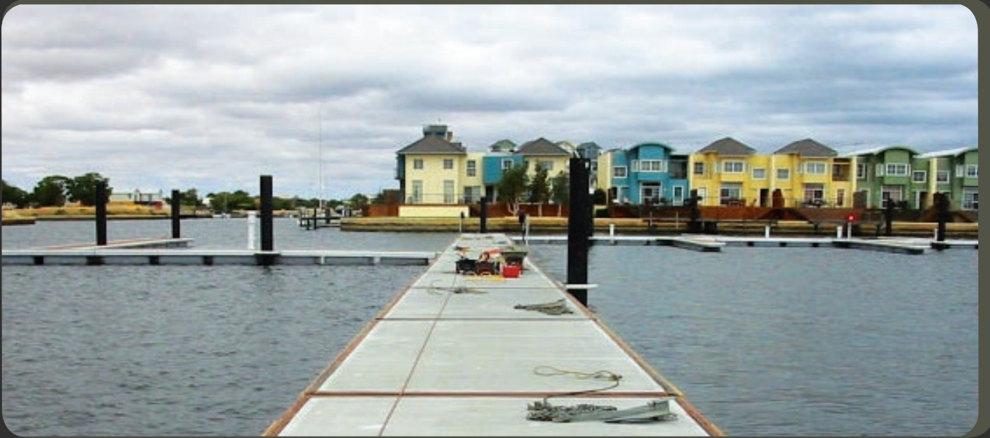
Main walkway at Port Geographe Marina
